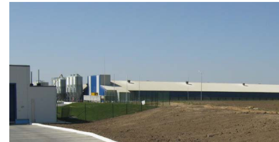
Rearing site. Construction of Stage 2
