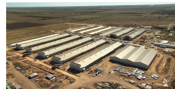
Industrial site. Construction of Stage 2
