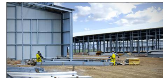
Industrial site. Construction of Stage 2
