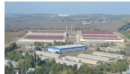
Construction of industrial site. Stage 2
