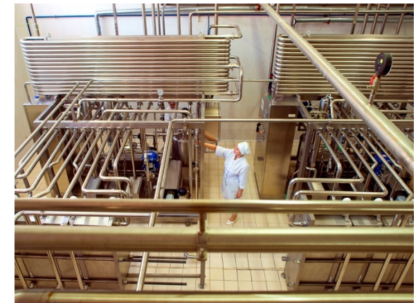
Imperovo Foods egg processing plant Cooling and reservation line
