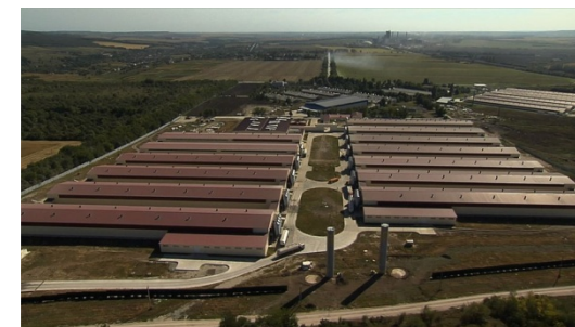
Industrial site. Stage 2
