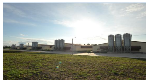
Avis. Rearing site (total capacity of 2.635 mn hens)
